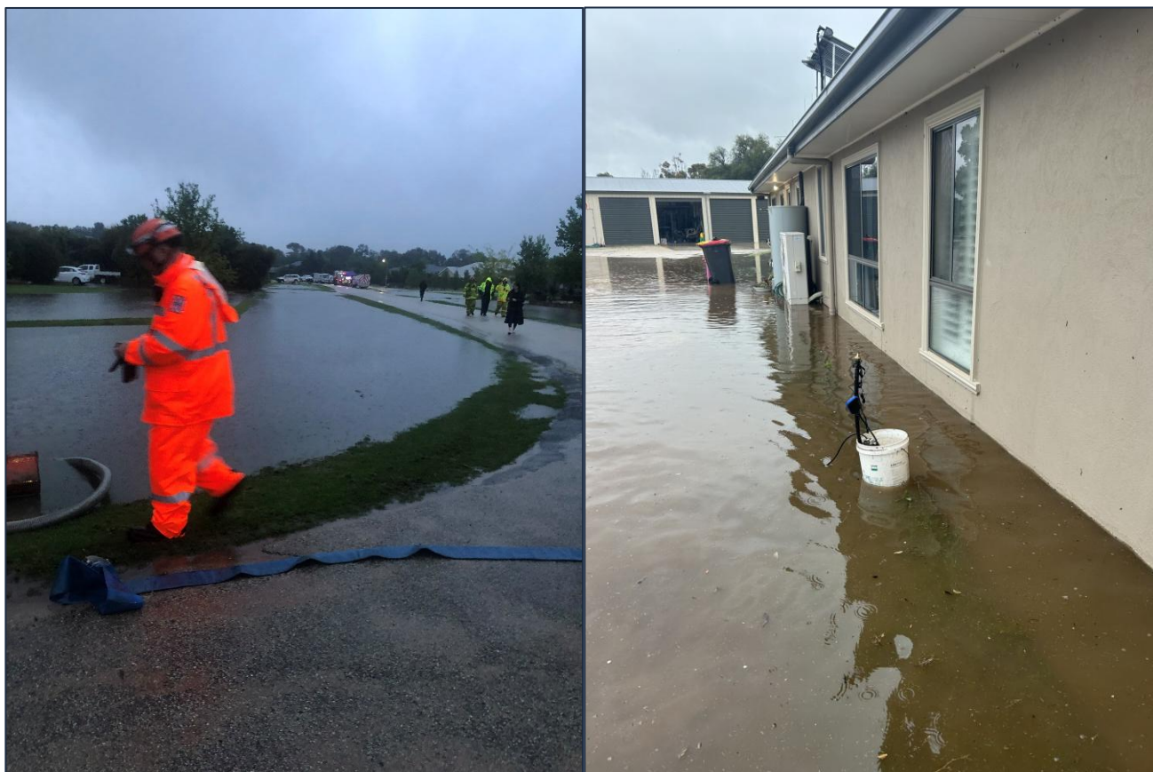
Figure 7-14 Photos Submitted by Community Members of Flooding on Charlie Gray Close
