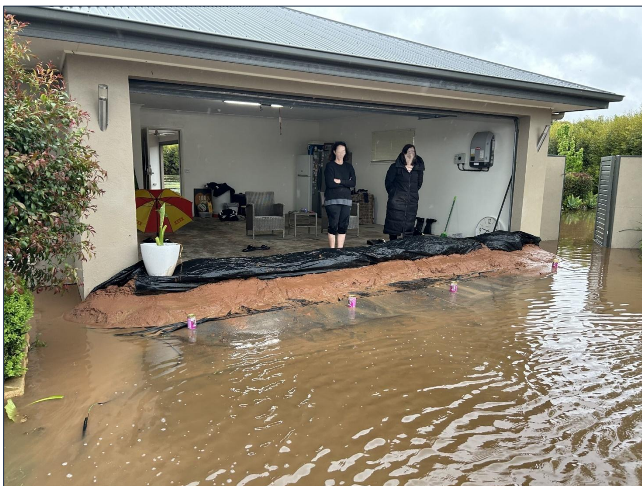
Figure 7-13 Flooded Residence and Temporary Flood Barrier on Charlie Gray Close
